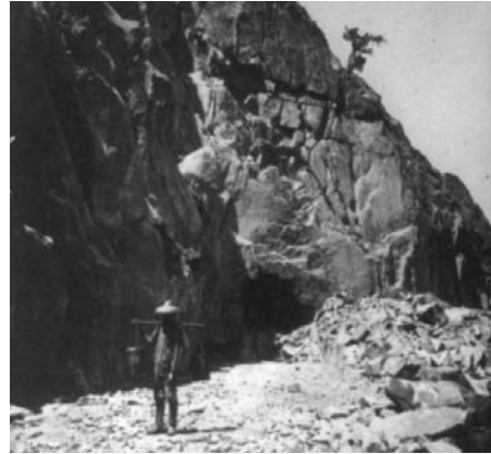
Photo: "Heading of east portal Tunnel No. 8" Hart, Alfred A. LOC 2005682948
